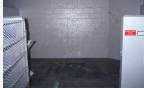
Stall with rubber mat over concrete floor
