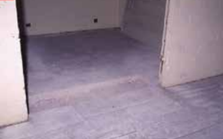
Stall with floor and walls made of concrete
