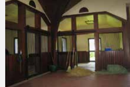
Stall with concrete floor and wooden walls
