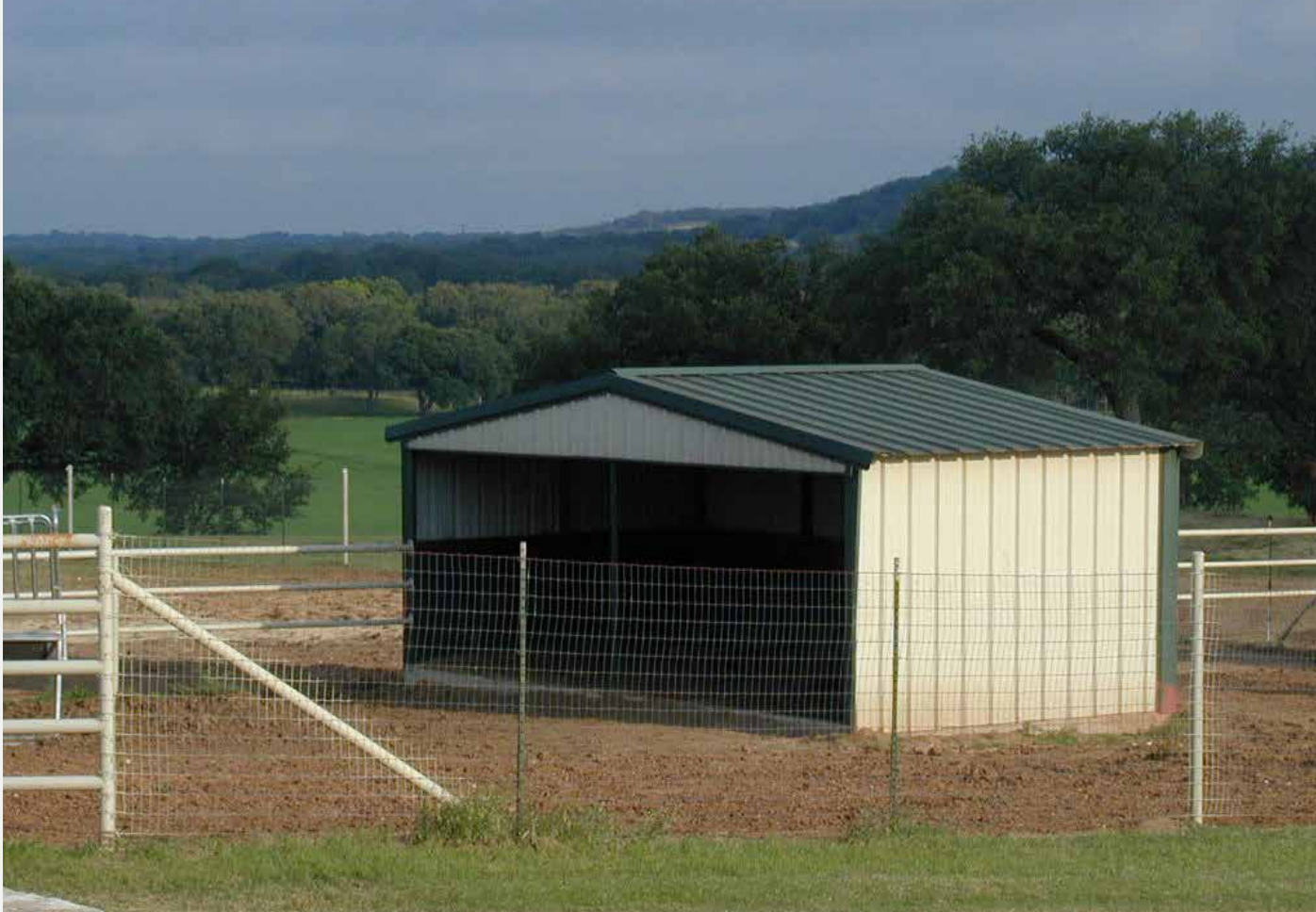
Isolation facility located away from main resident horse barn
